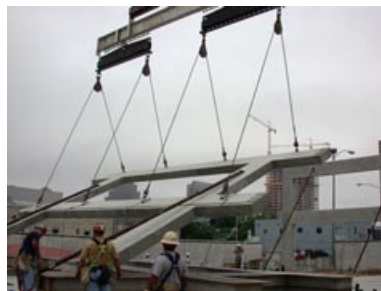
Cover Detail - south elevation with rain water collection tanks. TM 01 Detail - colored glass over entry ML 02 Stack-cast tilt-frames ready for installation. ML 03-06 Stack-cast tilt-frame installation. ML
