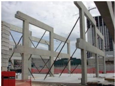
08 Tilt-frames in place. ML 09 Completed exposed frame – southwest corner. ML 10 Computer model tilt-frames. ML
