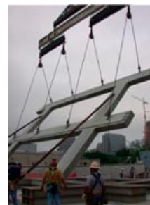
Cover Detail - south elevation with rain water collection tanks. TM 01 Detail - colored glass over entry ML 02 Stack-cast tilt-frames ready for installation. ML 03-06 Stack-cast tilt-frame installation. ML
