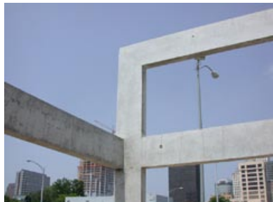
08 Tilt-frames in place. ML 09 Completed exposed frame – southwest corner. ML 10 Computer model tilt-frames. ML
