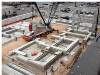
Cover Detail - south elevation with rain water collection tanks. TM 01 Detail - colored glass over entry ML 02 Stack-cast tilt-frames ready for installation. ML 03-06 Stack-cast tilt-frame installation. ML
