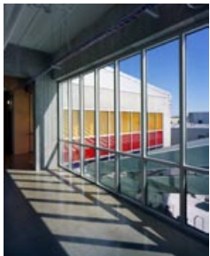
31 Entry windows seen □
